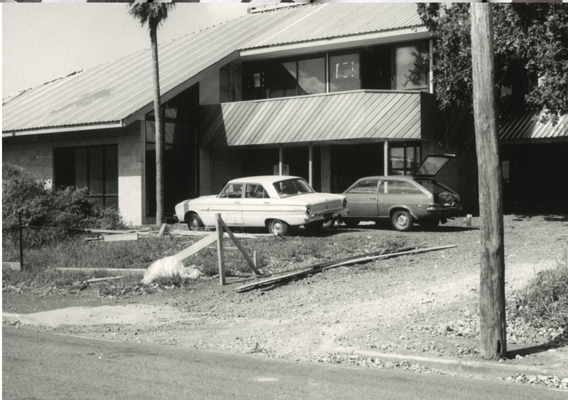
Mary Thomas Community Services Building under construction, formerly a tennis court for St Anne's School and car park for Takapuna Council. The St Annes building was demolished. Auckland Libraries Heritage Collections T1161
